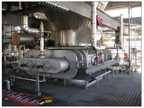
Shown are the open design and monorail system of the bottom unheading valve (Fig. 4).
