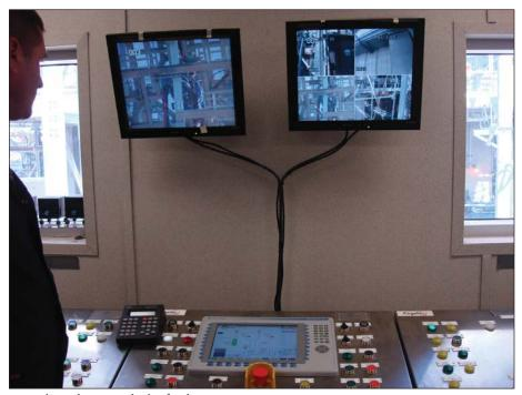
Fig. 5 shows the camera display for the operator.
